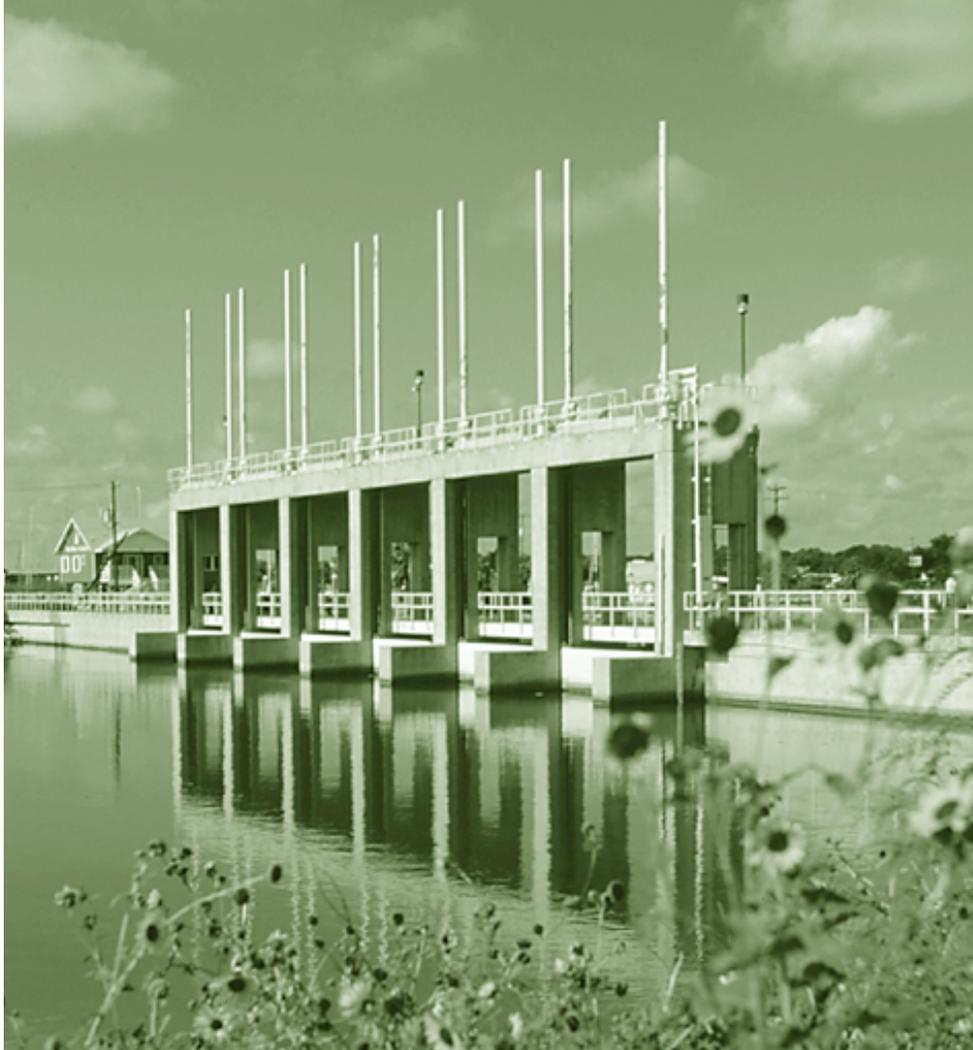
Each of the six, 20'x20' flood gates is driven by a 20 hp electric motor and provided with emergency power generation. The gates are opened when stormwater runoff causes the Clear Lake water level to exceed the Galveston Bay level.
