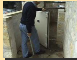
innovative flood gate
